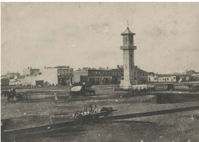
Fig. 1 View of Market Square and clock tower from Bright and Hitchcocks corner looking north east. Photograph by G. C. Wilmot, 1857. Geelong Heritage Centre GRS 2009/02050.
